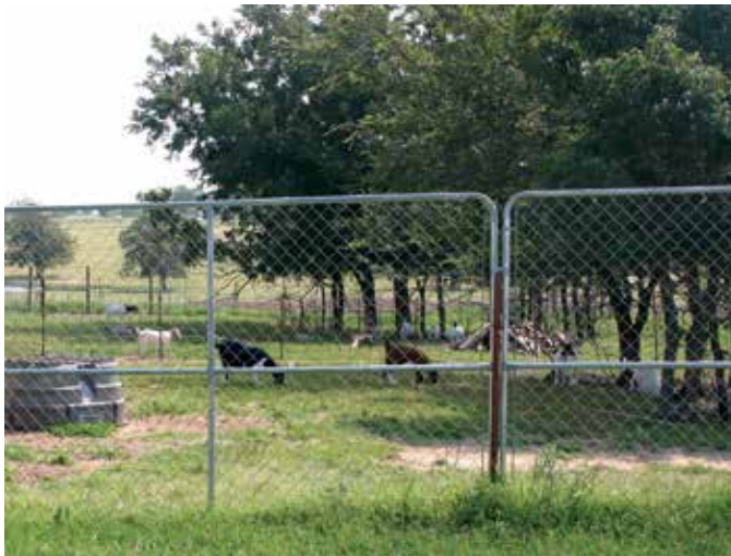
Figure 12-9. Chain link fencing.
