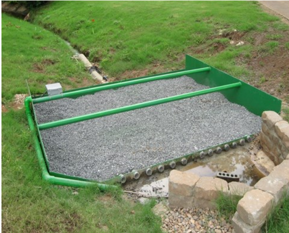
Phosphorus drainage filter installed at a golf course.
