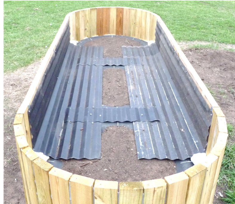
Completed bed ready to fill with growing medium.
