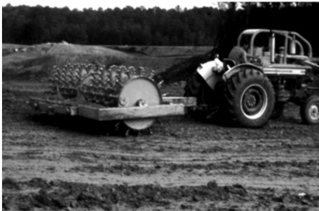
Figure 9. A sheepfoot roller can be used in compacting each lift during dam construction. Dozer tracks are a common alternative. Use of smooth rollers should be avoided. Image courtesy Alabama Cooperative Extension Service.
