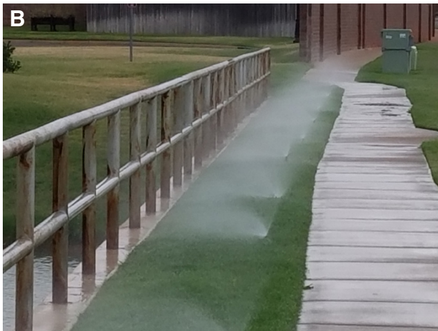
Figures 2a and 2b. High pressure in an irrigation system leads to misting and a reduction in irrigation efficiency. Photos courtesy of Oklahoma City Utilities Department.
