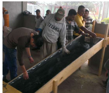
INSTALLING LATH
