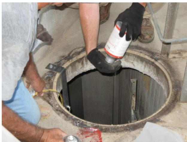
**Figure 5. Applying phosphine pellets in a concrete silo.**
