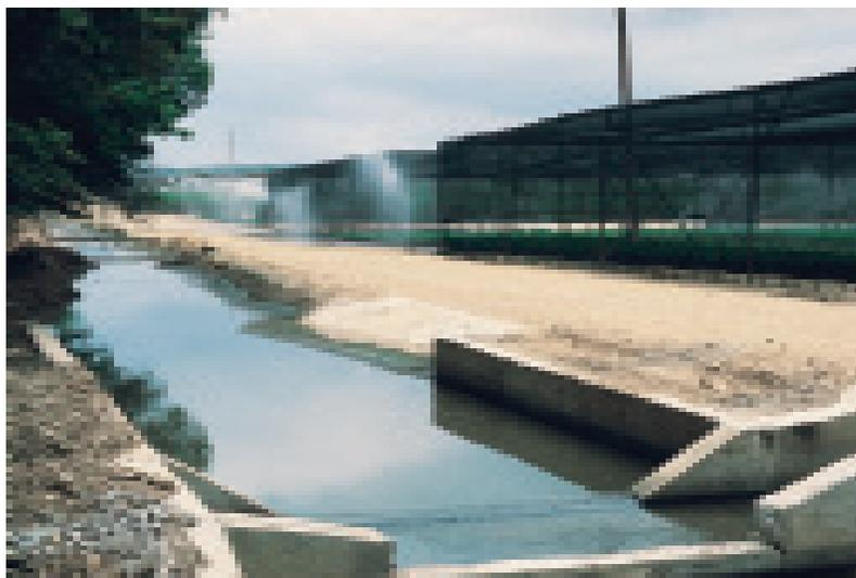
In a capture and recycle system, irrigation runoff from nursery beds and houses in production areas is collected by a system of channels or ditches leading to retention basins.
