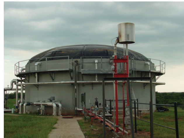
Figure 12. ASBR digester located on the Oklahoma State University Swine Research and Education Center.
