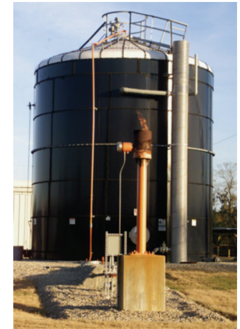
Figure 8. Fixed Film Digester located on the University of Florida Dairy Research Farm (Photo courtesy of Ann Wilkie, University of Florida).
