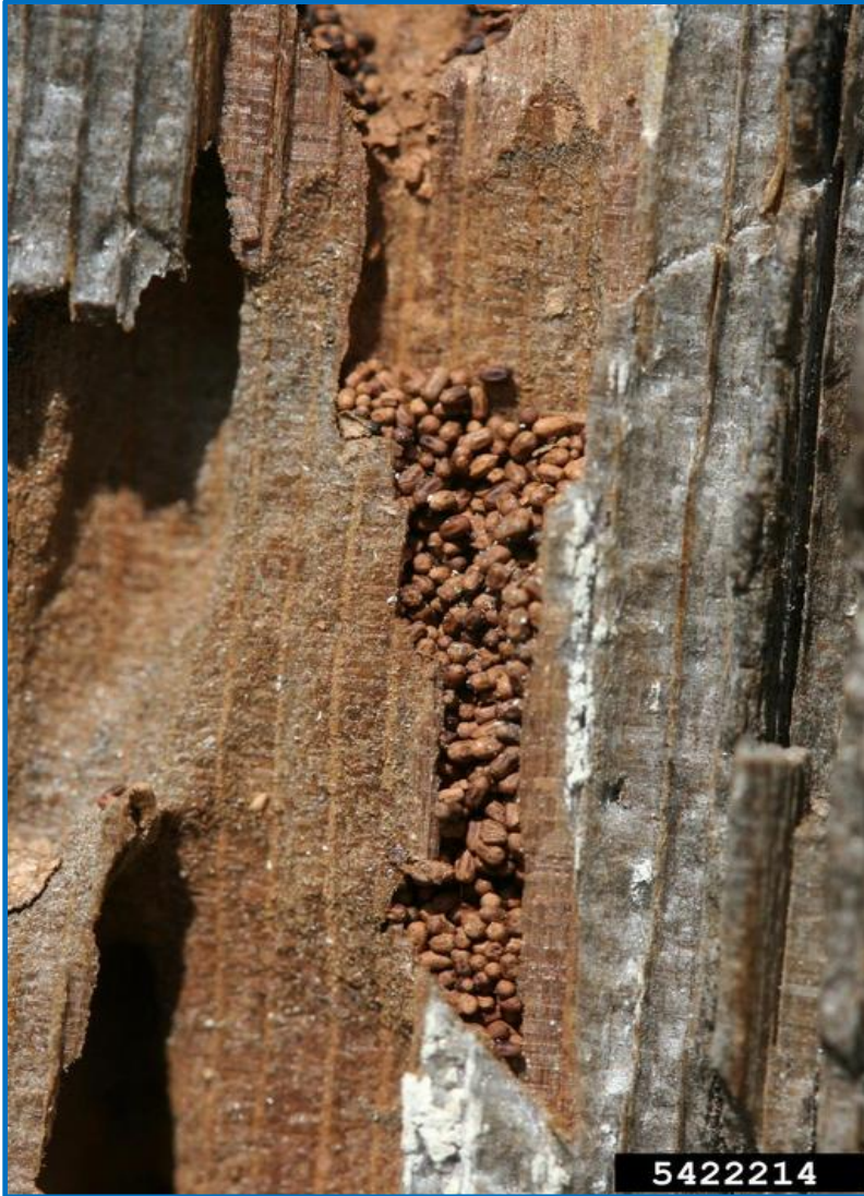
Fig. 10. Drywood termite fecal pellets (frass) stored in a hollowed-out gallery in a wood board. Note that galleries are not packed with mud like found with subterranean termites.
