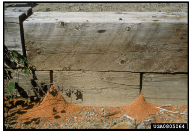
Figure 4. Evidence of carpenter ant activity. Excavated sawdust discarded from a nesting site. [Photo courtesy Edward H. Holsten, Bugwood.org]
