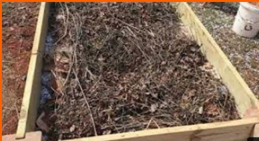
Simple Raised Bed Garden Construction
